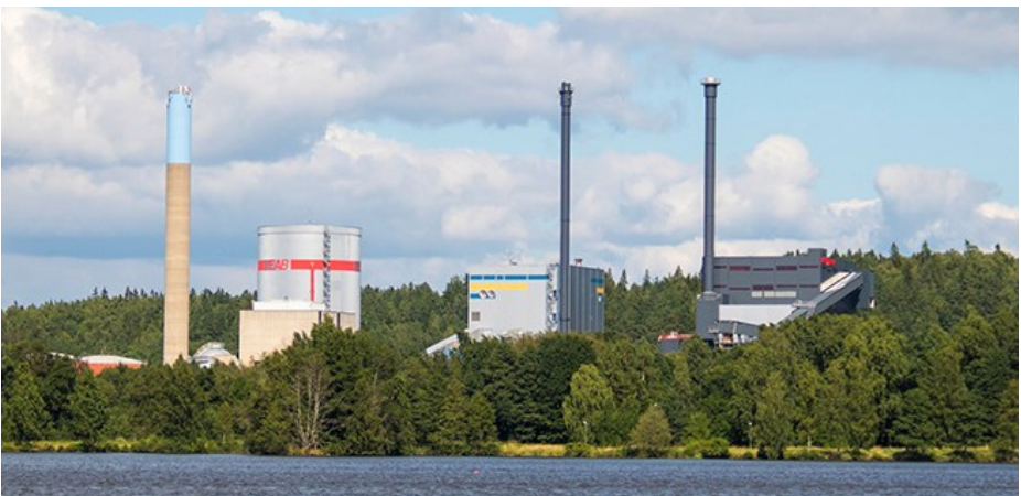
Sandvik II, biomass combined heat and power plant
